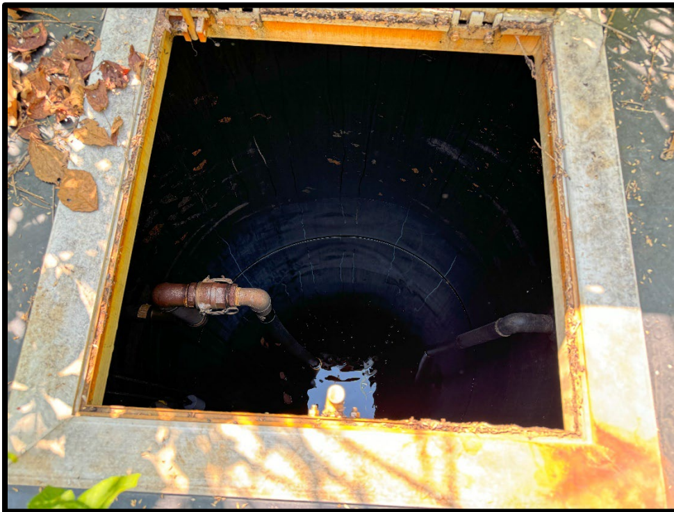
Photograph 4: View of VLCS-2 sump at 1/4 – 1/3 capacity.
