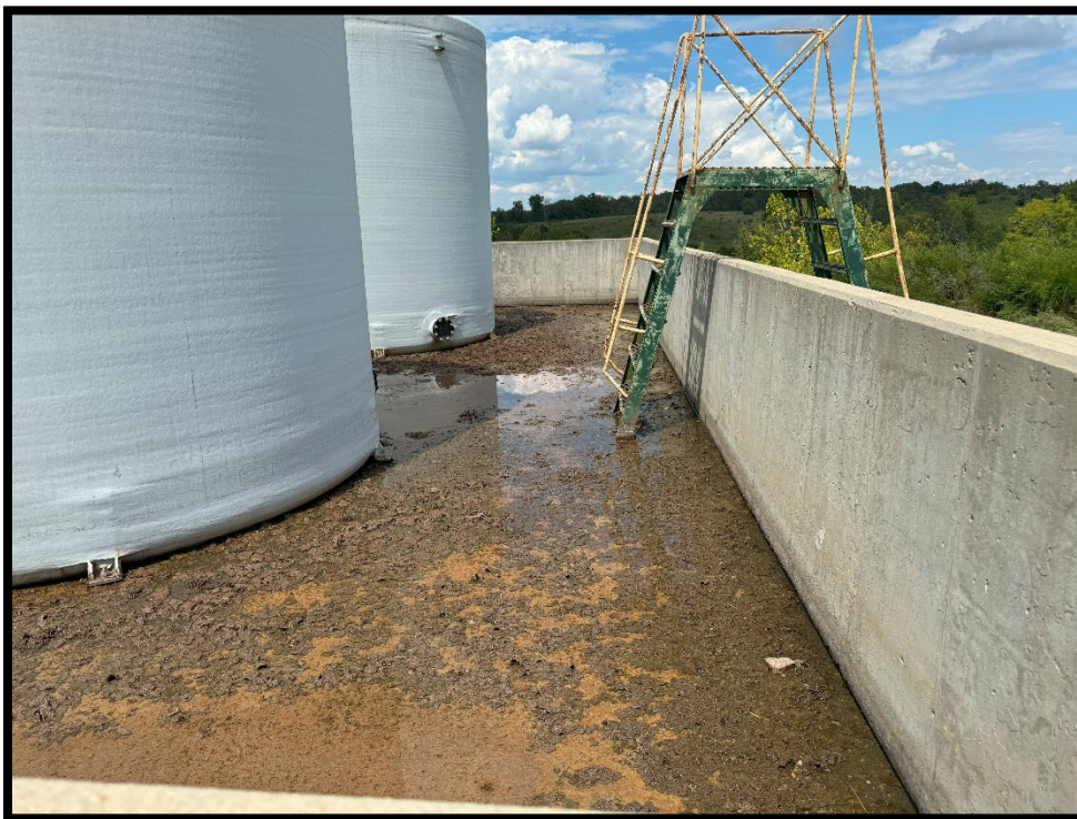
Photograph 6: View north of minimal stormwater in leachate tank secondary containment.
