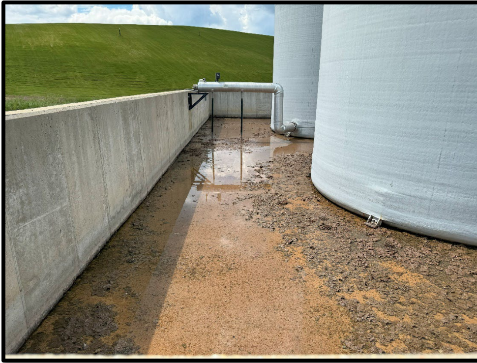
Photograph 5: View west of minimal stormwater in leachate tank secondary containment.
