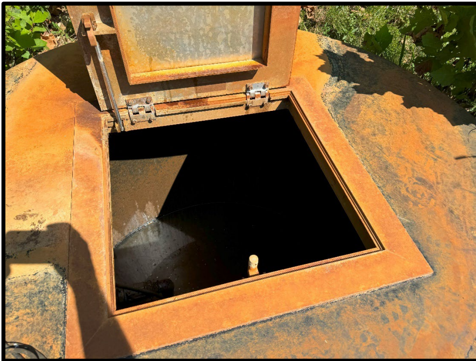
Photograph 2: View of VLCS-1 sump at 1/2 - 2/3 capacity.
